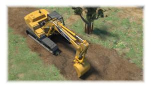
Sometimes contractors may use a borrow pit (also called a sand box). A borrow pit is an area where soil, sand or gravel (material) is dug out to be used in another area. Sometimes the borrow pit will become the drains, or water catchment areas at the end of the work.
