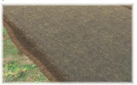
Once the subbase is at the right thickness and is compacted properly, trucks deliver the course road base. The road base is built up in many layers. Water trucks may wet down the road base if it helps the roller/compactor compact the base.
