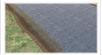
If asphalt is being laid, more layers will go on top of the road base. There will be an asphalt base course, then a binder course, and finally, a surface course.
