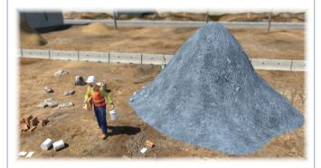
When you fill out a stockpile, start by filling the area closest to the back of the stockpile area.
