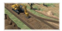
As the operator shapes the ground, they will usually create drainage at the sides of the road area. They will also make sure there is enough fall (scope) on the road so that water drains away from the road.
