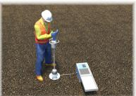
Many layers of the ground material are built up. This is called the subgrade. Each layer is compacted and tested.
