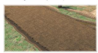
Trucks then deliver subbase. Haul trucks or tip trucks sometimes tip the subbase, and front end loaders spread it.
